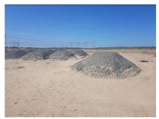
Image 13: Stockpiling of aggregate.
