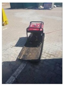
Image 2: Generator coupled with a drip tray.
